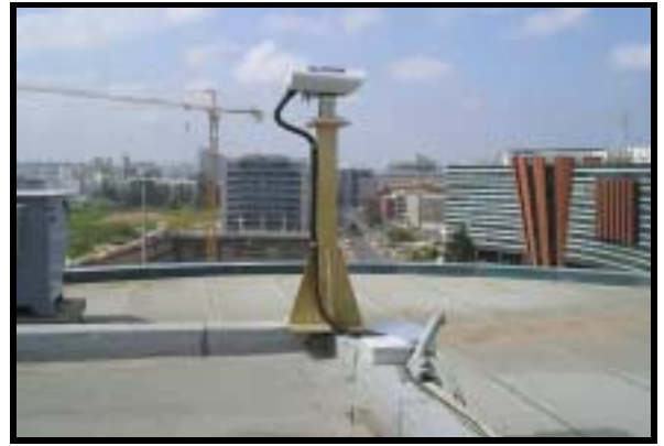
Figure 2.7: Floor Pedestal Mounting (using JMP and M015C)
